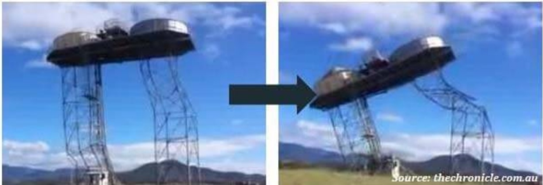
Buckling of a water-reservoir's columns
